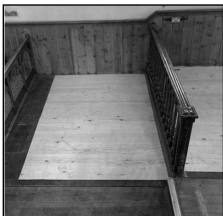
New floor timbers in St Ethelbert's Church, Thurton
